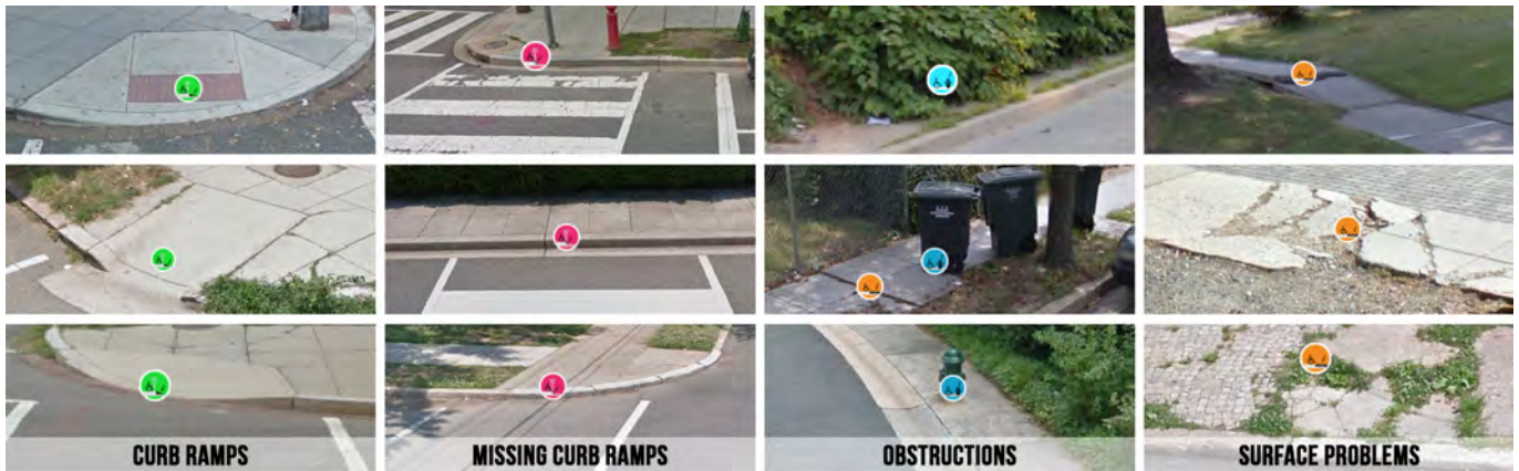
Figure 1: Examples of the four label types used to train and test our deep learning models for semi-automatic sidewalk assessment: curb ramps , missing curb ramps , obstructions , and surface problems . Figure adapted from Project Sidewalk [55].
